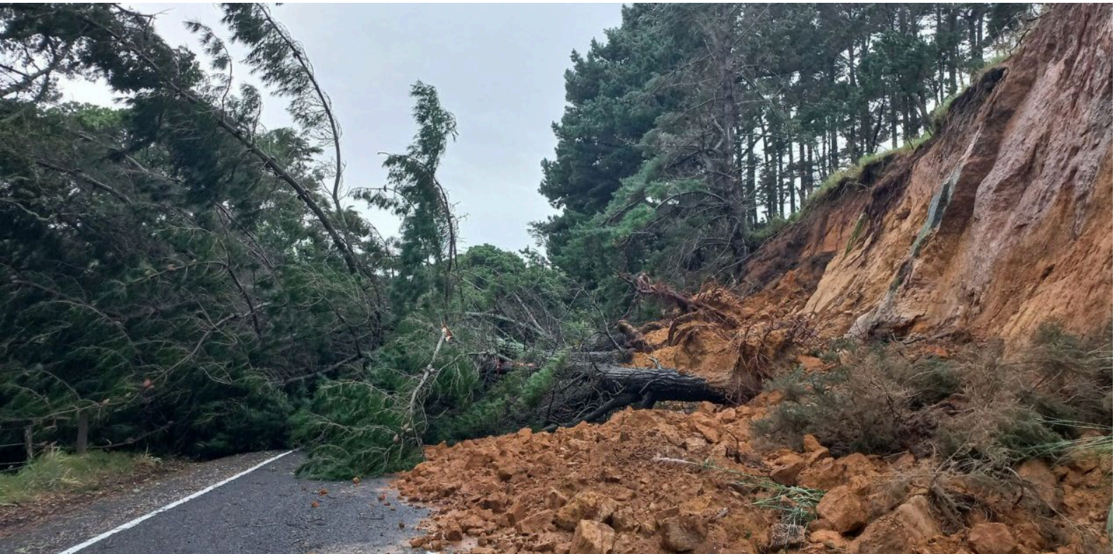
Landslide impacting road transport
